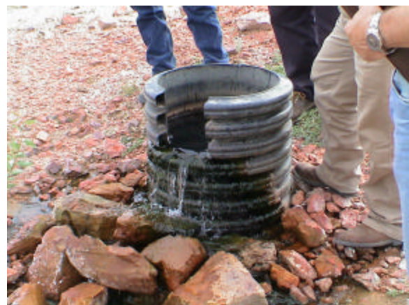
Direct Surface Discharge Location
