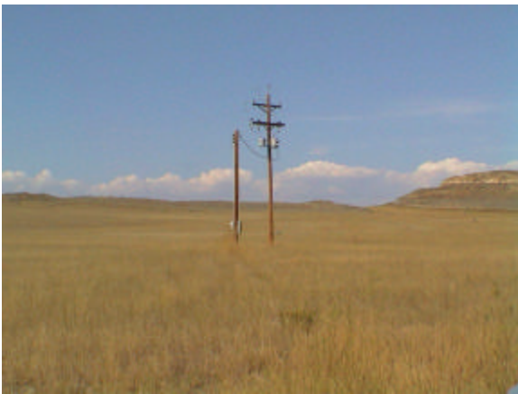
Underground Utilities for CBM Facilities Connected to Existing Power Lines
